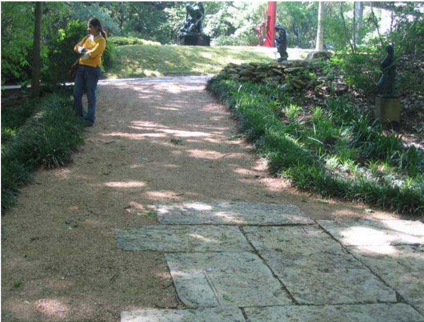
This pathway originally was paved all over, however the edges were uneven and during rainy season the stones became very slippery making it difficult for wheelchairs. Part of the paving has been stripped down and has been converted into gravel pathway for the convenience of people on wheelchair.
